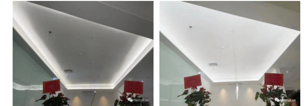
Illumination effect of light strip without light distribution
