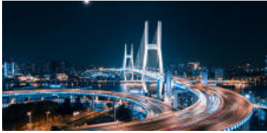
ROAD & OUTDOOR LIGHTING
